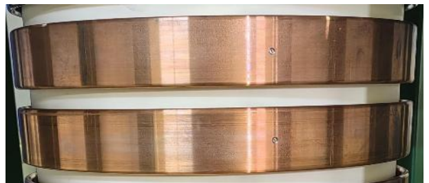
Fig.4. Smooth surface of the lower gas part of the individual insulator with shielding rings.
